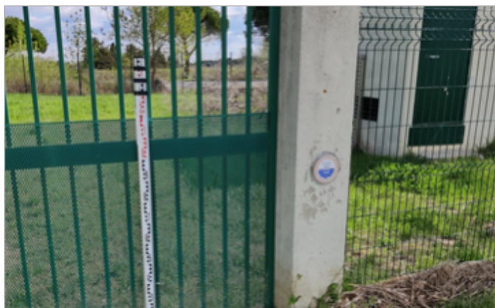
pilier station pompage
