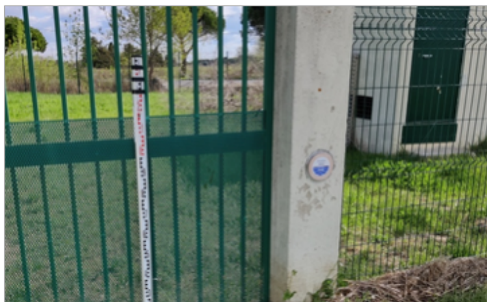
pilier station pompage
